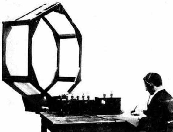
A wireless telegraphy receiver used in France between 1925 and 1928 (Photo: Thomson-CSF)
